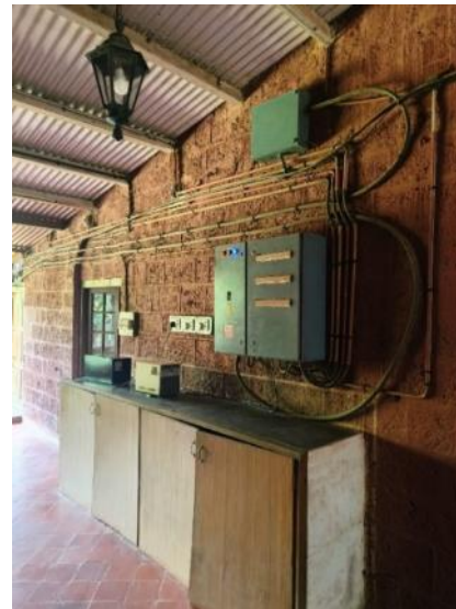
Removing redundant cables and re-routing
