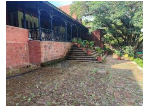
Repairs of steps from Patio & doing laterite paving
