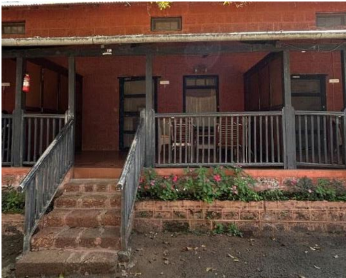
Existing railing with Wooden Balustrades
