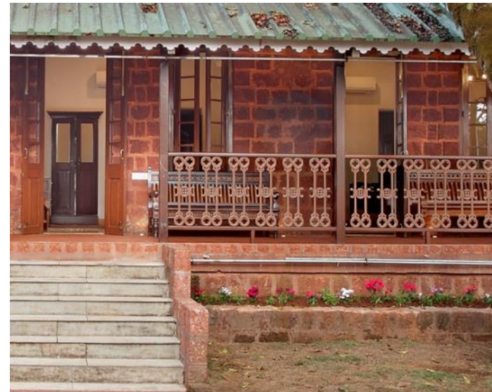
Proposed railing with Cast Iron Balustrades
