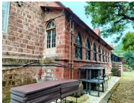
Re-routing the electrical cables in underground fashion and not on the structure
